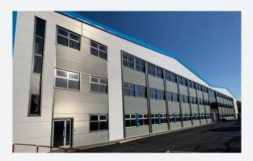
Due to the close proximity to the Airports radar, the Southern elevation external materials had to be non-metallic with the window / fenestration installed at a 5 degree angle to the main elevation.
